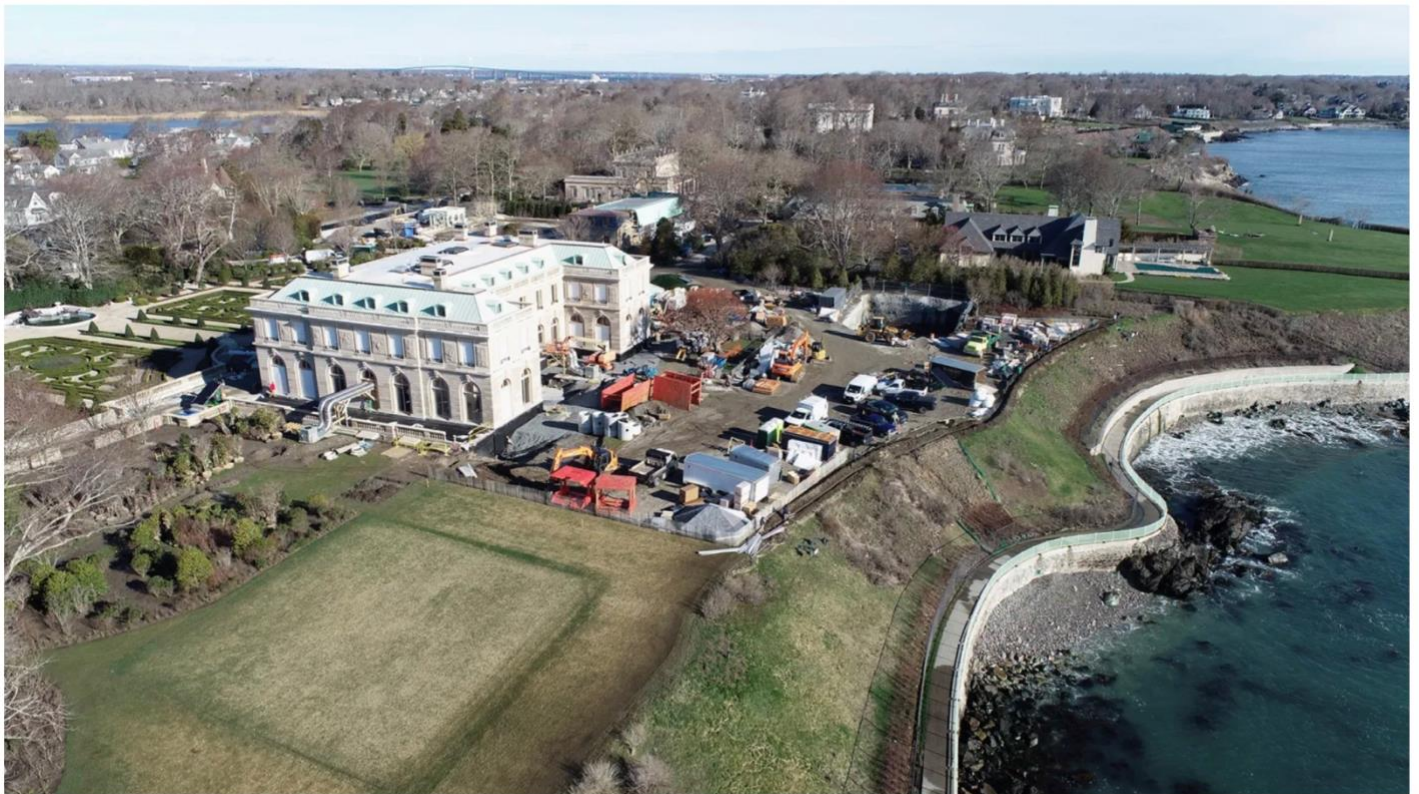
Miramar under construction Courtesy photo
