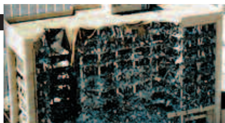
Murrah Federal Building
