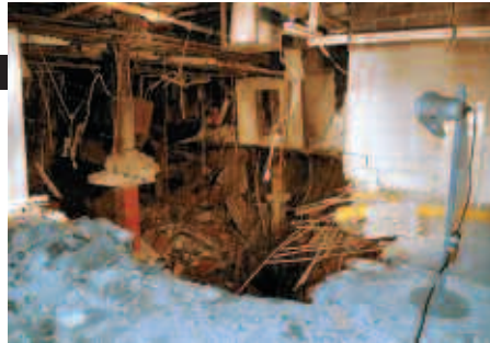
Bomb damage at the WTC
